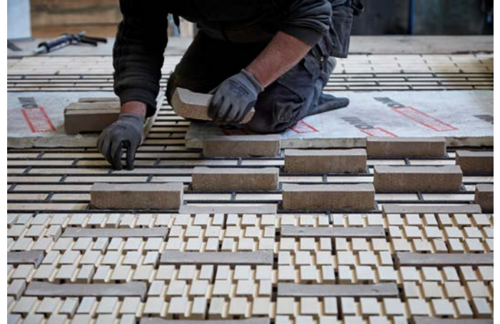
Stretcher bond brickwork being laid into mold
