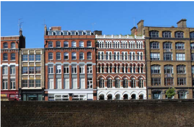
Farringdon Road streetscape
