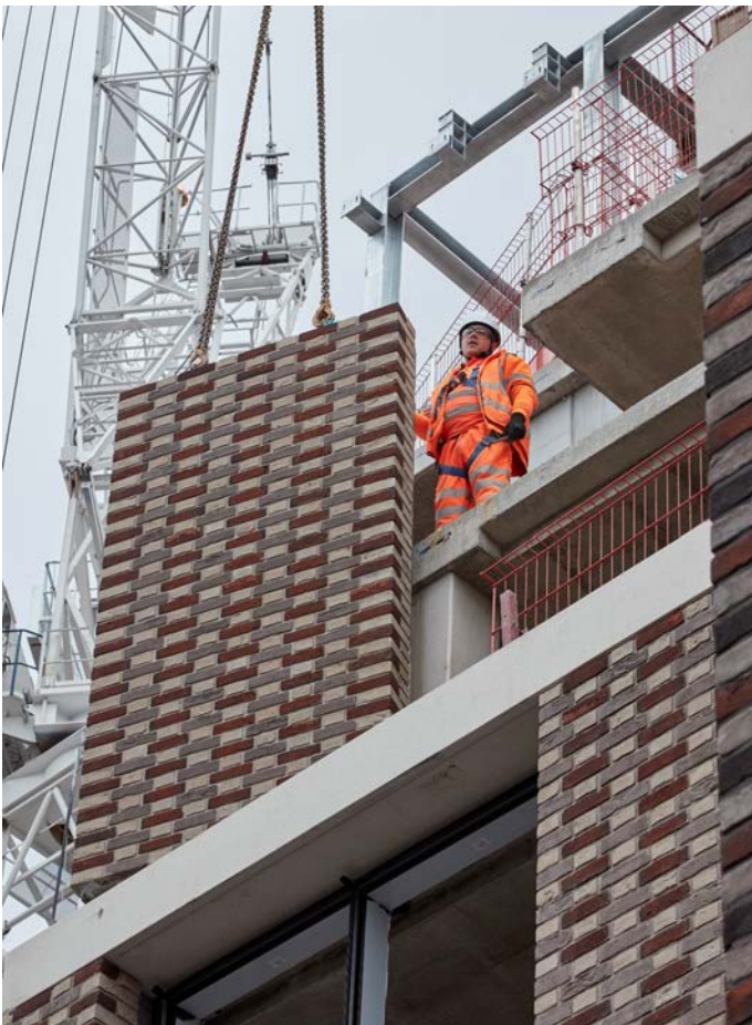
Flemish bond panel being installed on site
