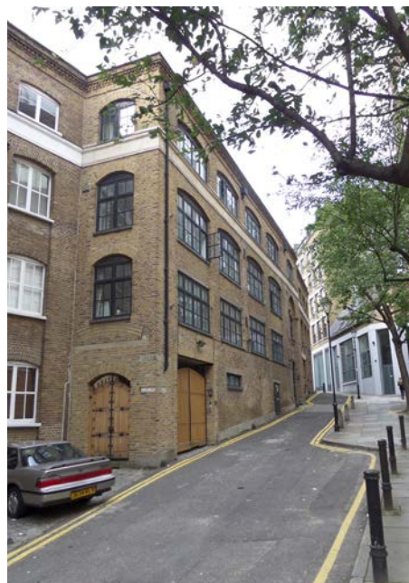
View of Crawford Passage looking north
