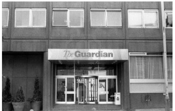
The Guardian building, detail of previous main entrance
